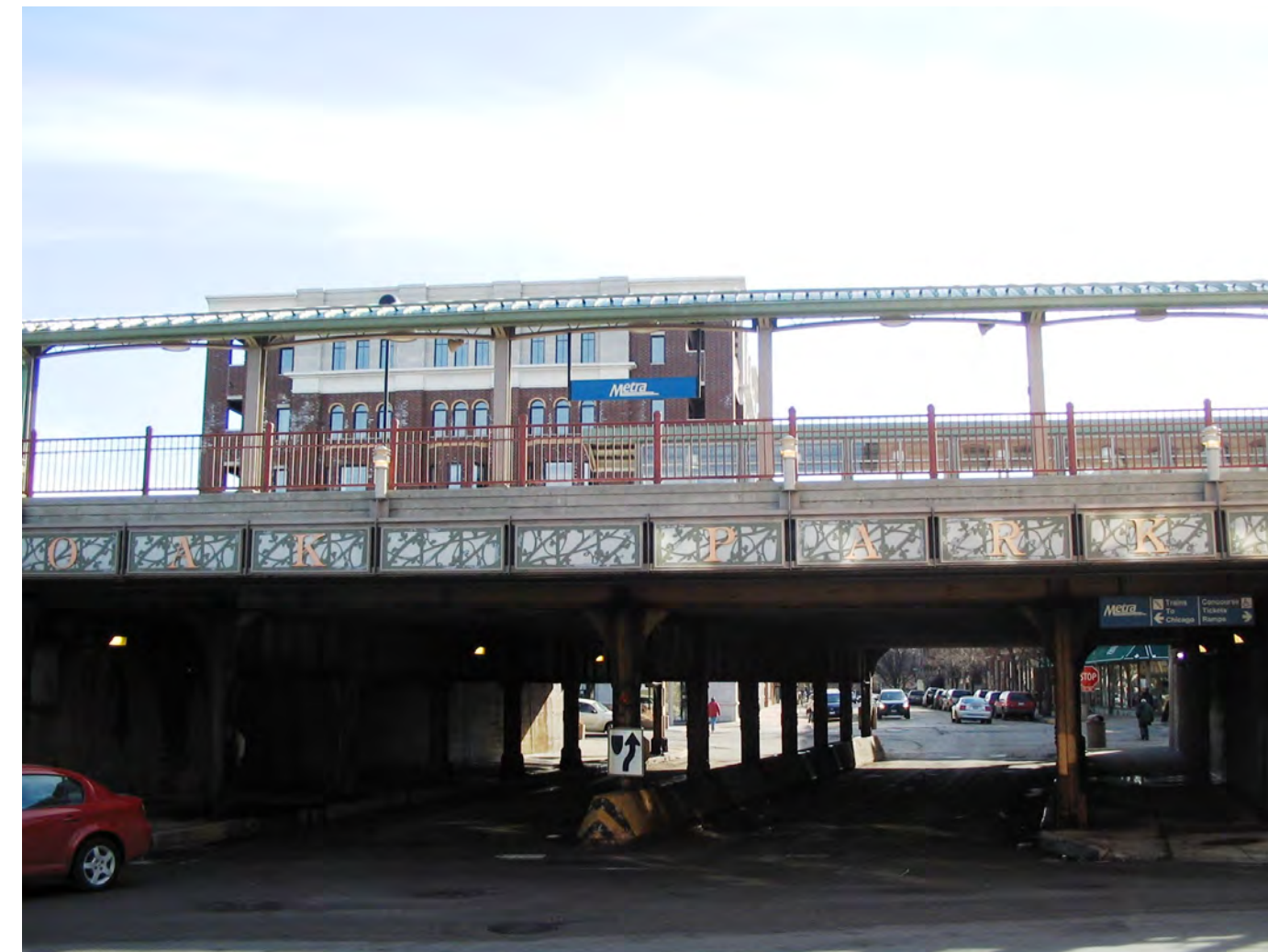
Example of facade and railing enhancements on a railroad structure (Oak Park Metra Station)
