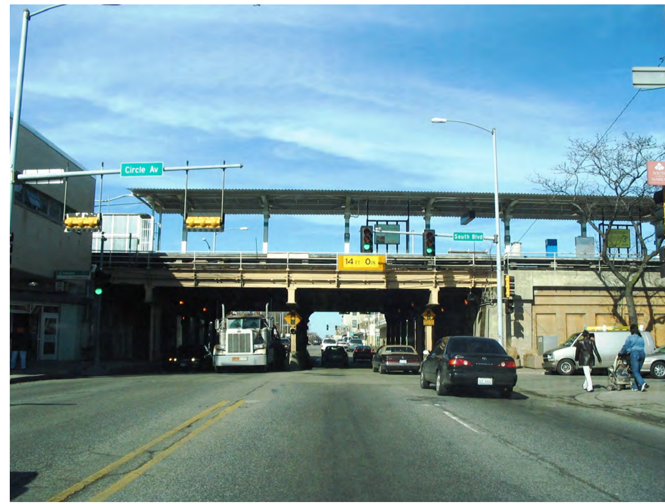
Harlem Avenue underpass looking north
