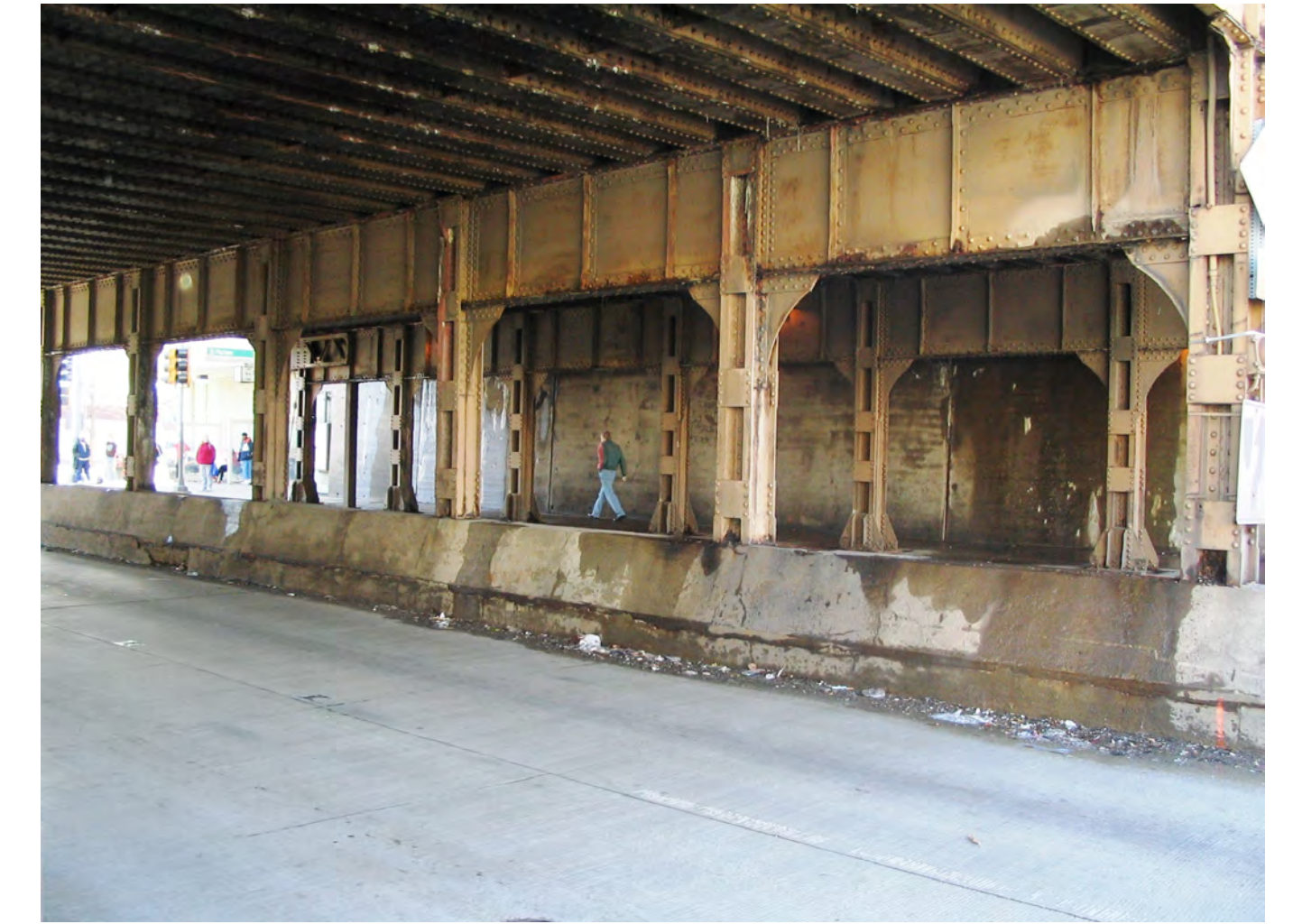
Underpass piers and columns
